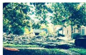
Demolished in one day!
